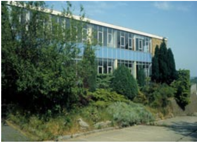
In 1983 these 20-year-old, Architect-designed buildings, had so little strength the floor sagged under filing-cabinets. There was no heat or sound insulation and no sunscreening.
