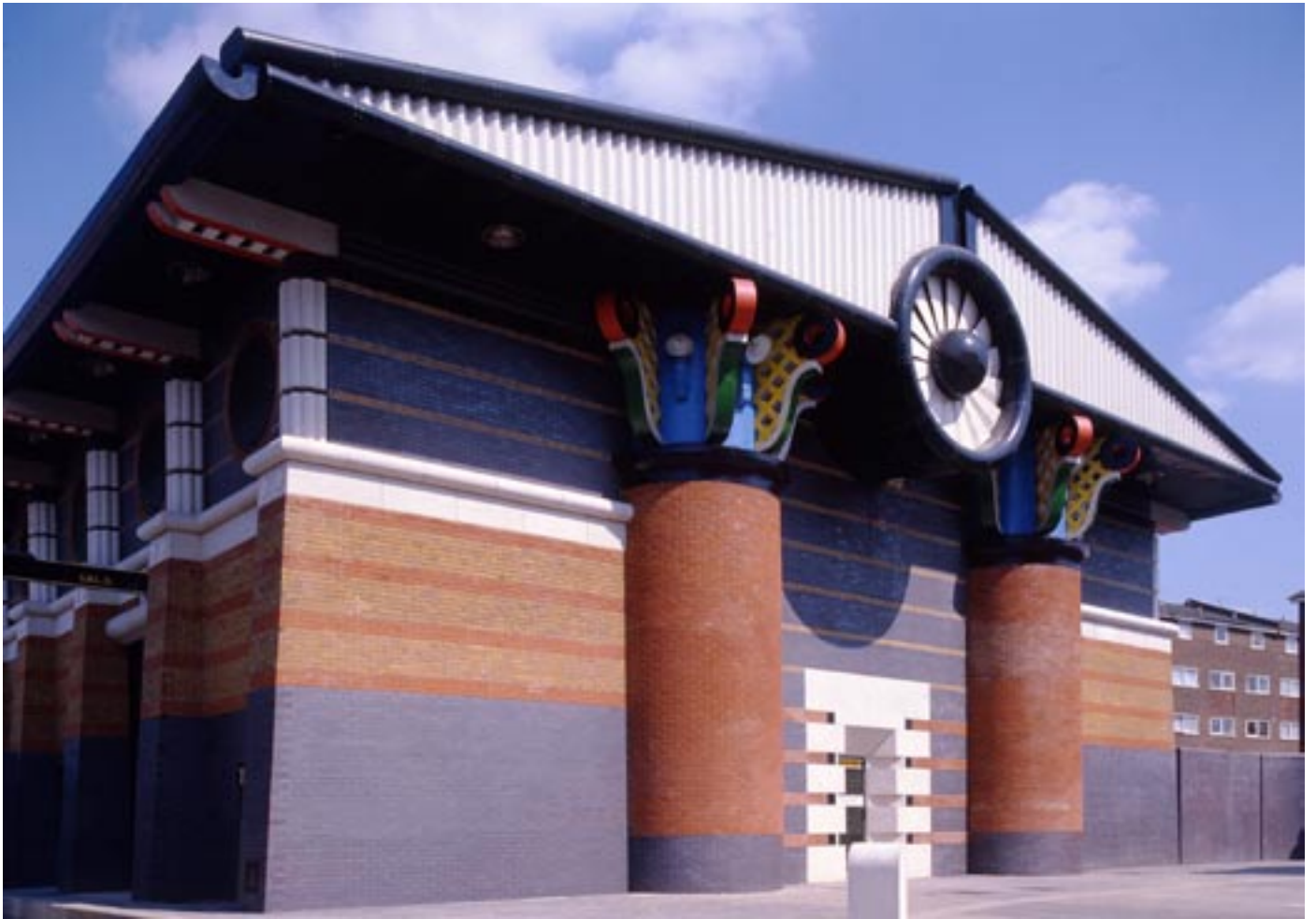
Isle of Dogs: Stormwater Overflow Pumping Station. Required structural life - 100 years. Physical function - to save the Isle of dogs from being flooded with raw sewage when it rains in Mayfair. A monument to summer storms - opened on a Thors-day.
