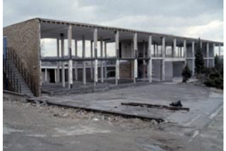
Keeping their structural frame, drainage and landscaping allowed four months to be cut from the construction timeline. So they were stripped-down and re-clad.
